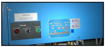
The HES Series control panel was upgraded to a Hoffman enclosure is 2010. The serial number nameplate is located on the upper right corner of the control panel door as shown below.
